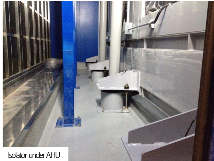
Isolator under Rotating Machine
